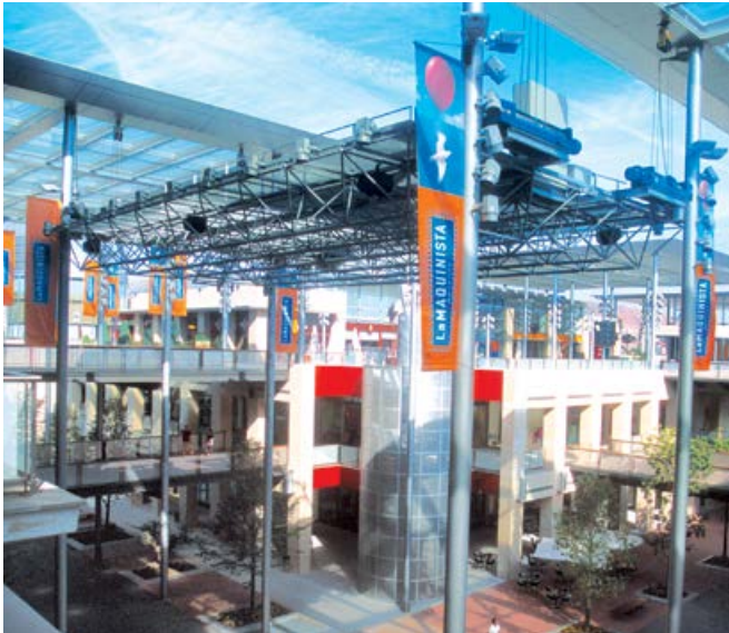
Synchronised DH hoist units lift and lower a roof segment in a shopping centre
